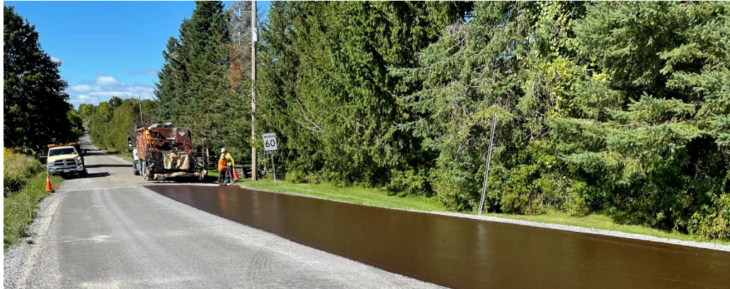
Cartwright West ¼ Line Rehabilitation
