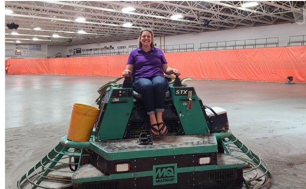
Scugog Community Recreation Centre Pad 1 Refrigeration Pipes Replacement
