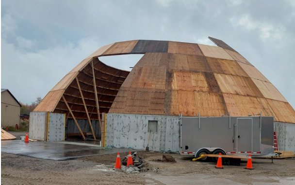
Port Perry Depot Sand Dome under Construction
