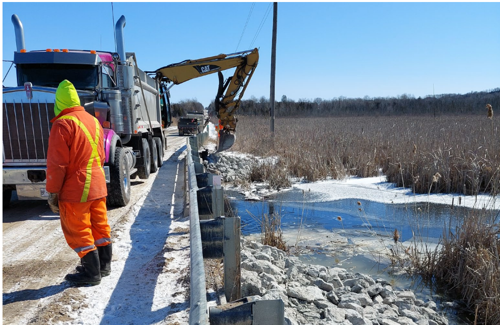
PWIS Team Undertaking Bridge Repairs on Scugog Line 12
