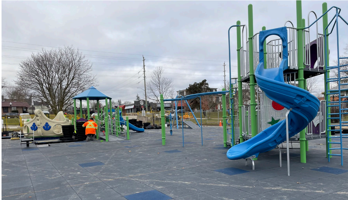
New Junior and Senior Playgrounds at Palmer Park Being Installed
