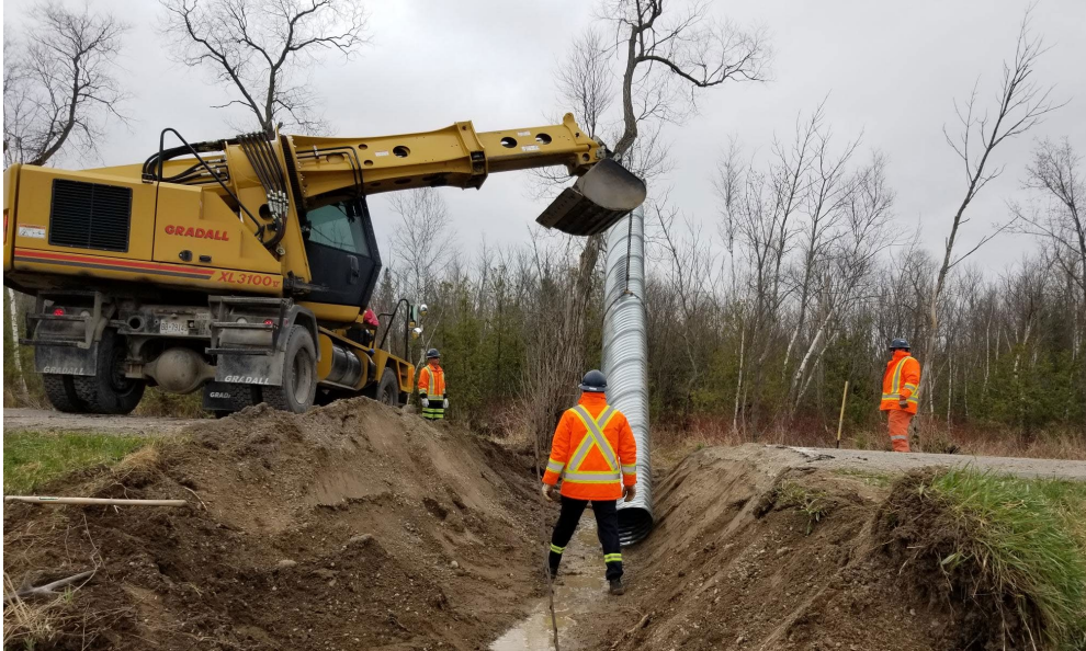
PWIS Team Replacing Cross Culvert
