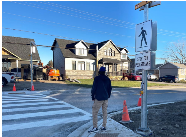
New Pedestrian Crossover on Old Simcoe Road
