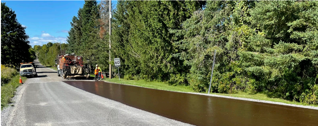
Cartwright West ¼ Line Rehabilitation
