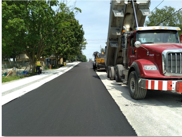
Major Street Reconstruction
