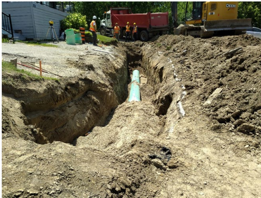
Portview Road Drainage Repairs
