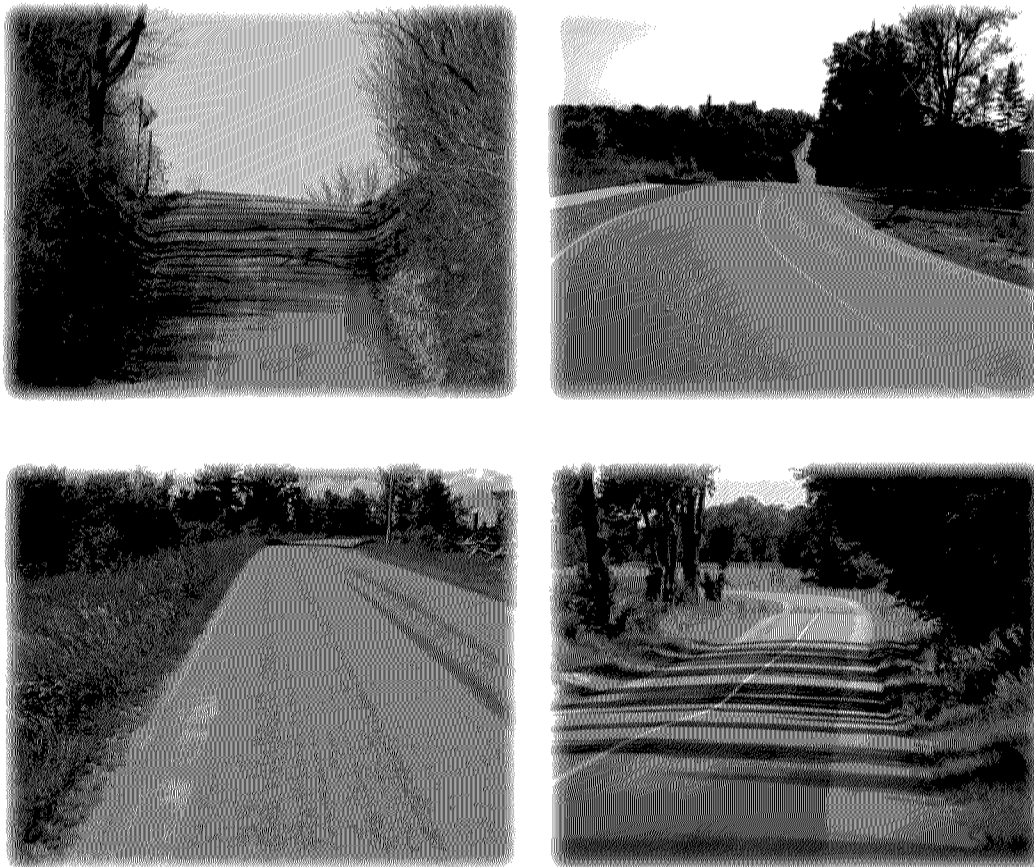
Figure 6.2: Potentially Substandard Vertical and Horizontal Alignment
