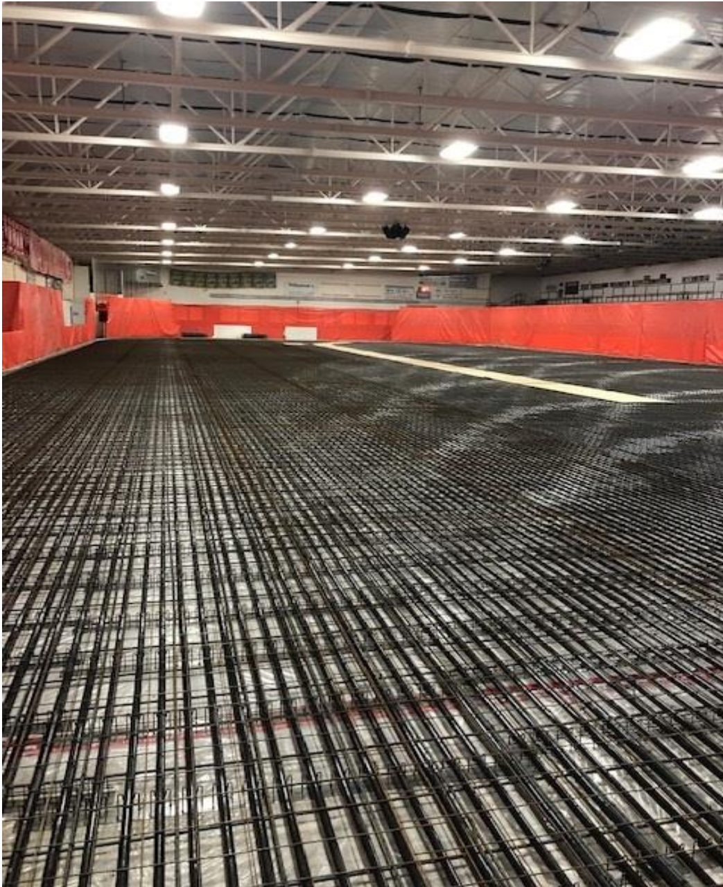
SCRC Pad 1 brine pipes and headers replacement
